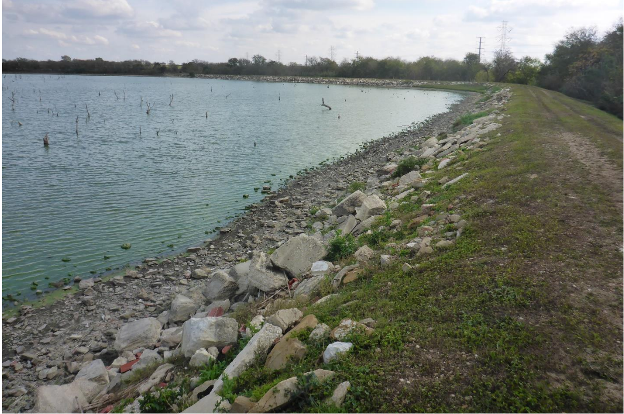
Photo 3: Upstream Embankment Slope
