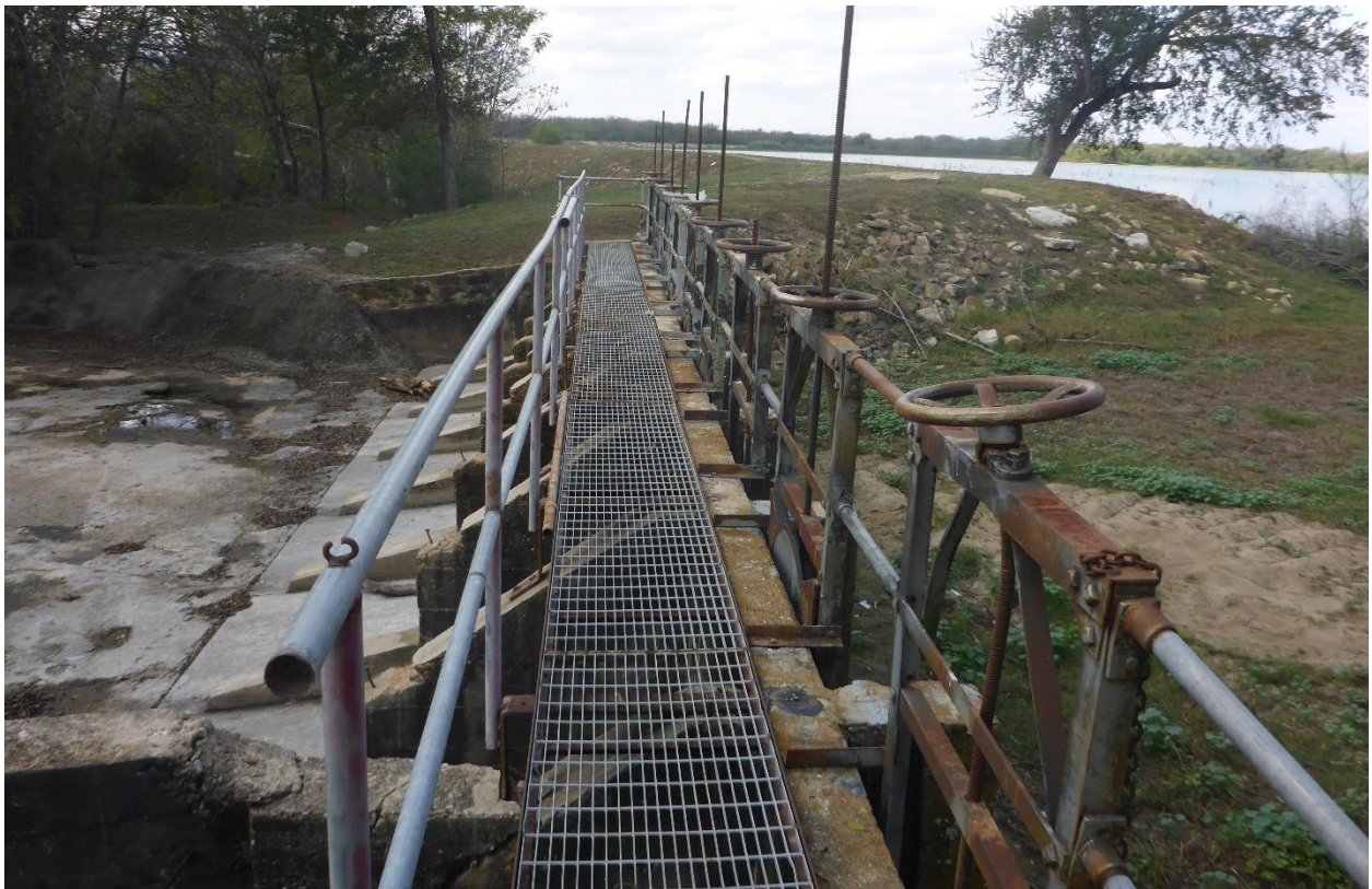
Photo 12: Spillway Bulkhead Catwalk and Gate Handwheels
