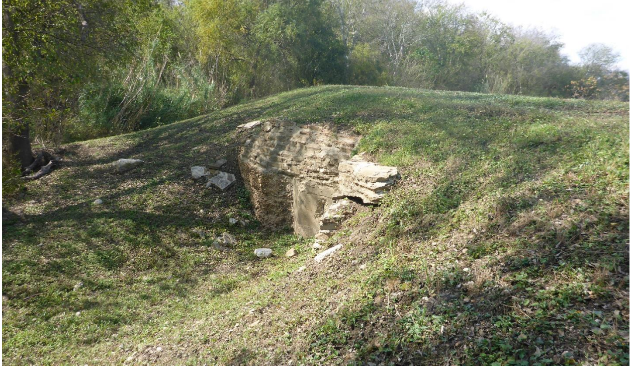
Photo 5: Headwall Structure on Downstream Slope
