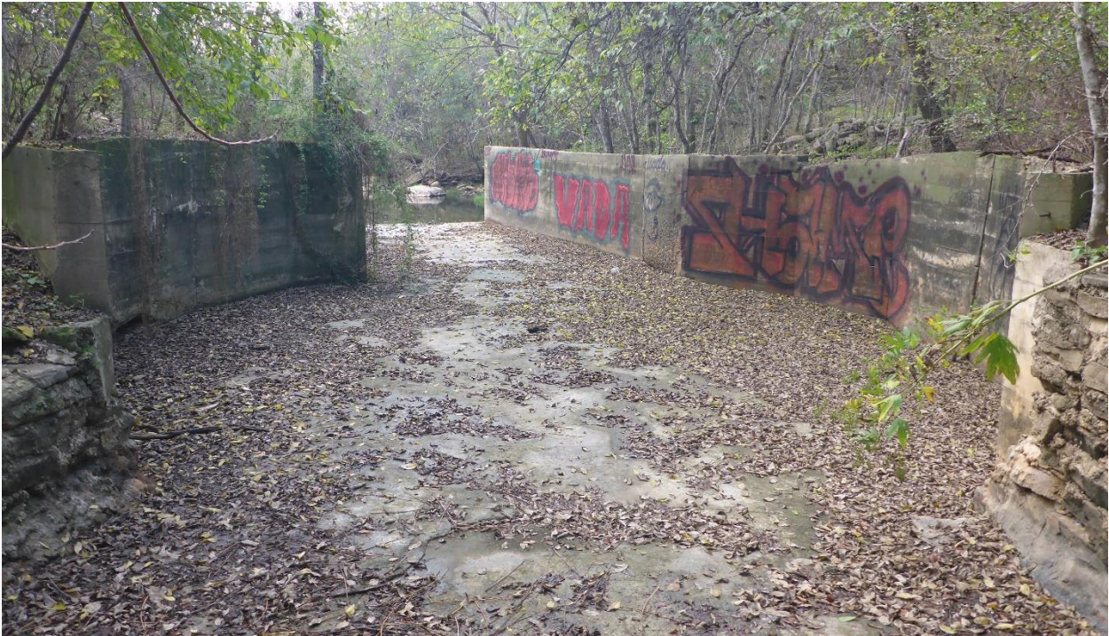
Photo 16: Spillway Channel Looking Downstream
