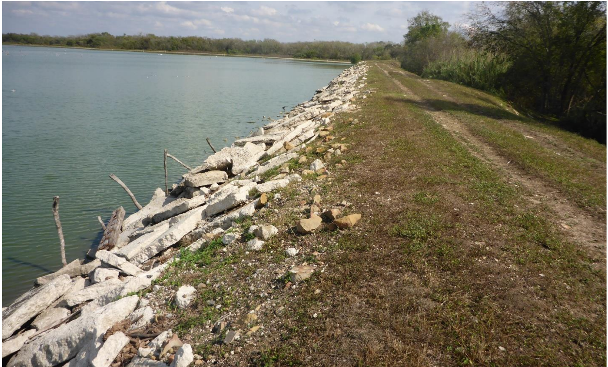
Photo 6: Upstream Embankment Slope
