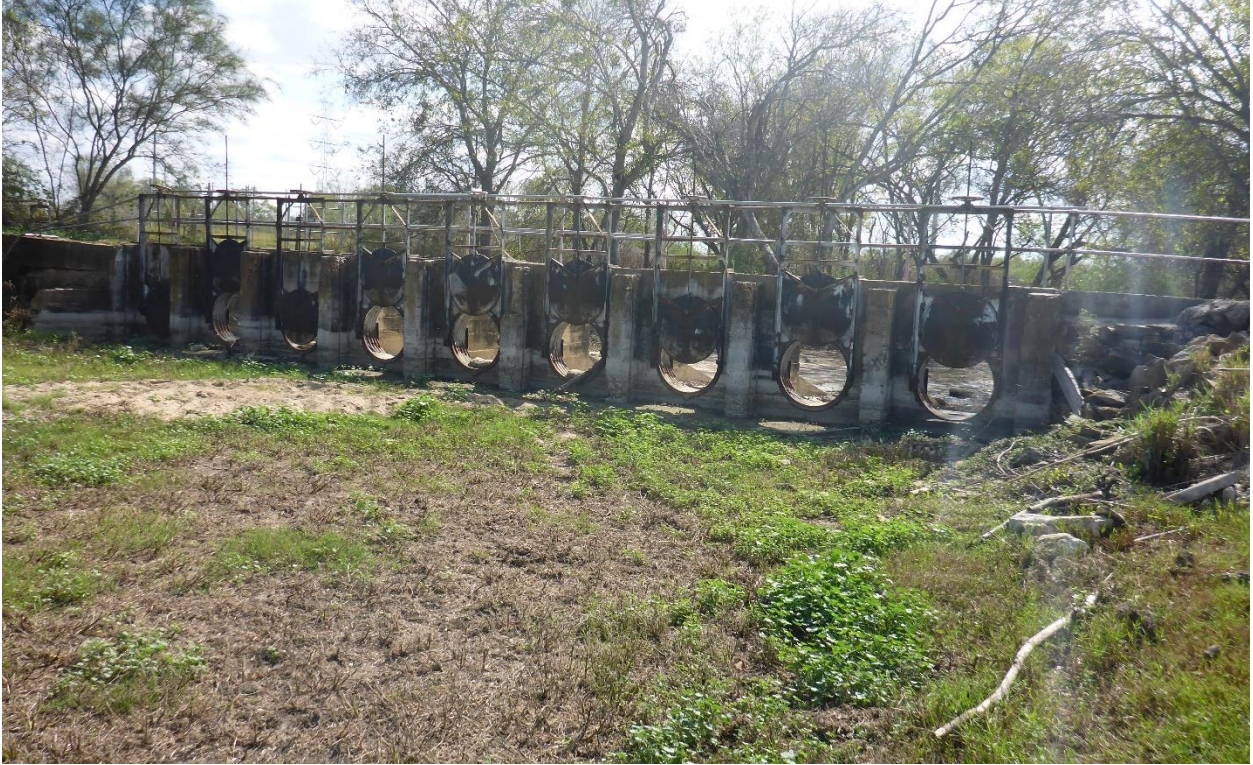
Photo 9: Spillway Upstream Face and Gates
