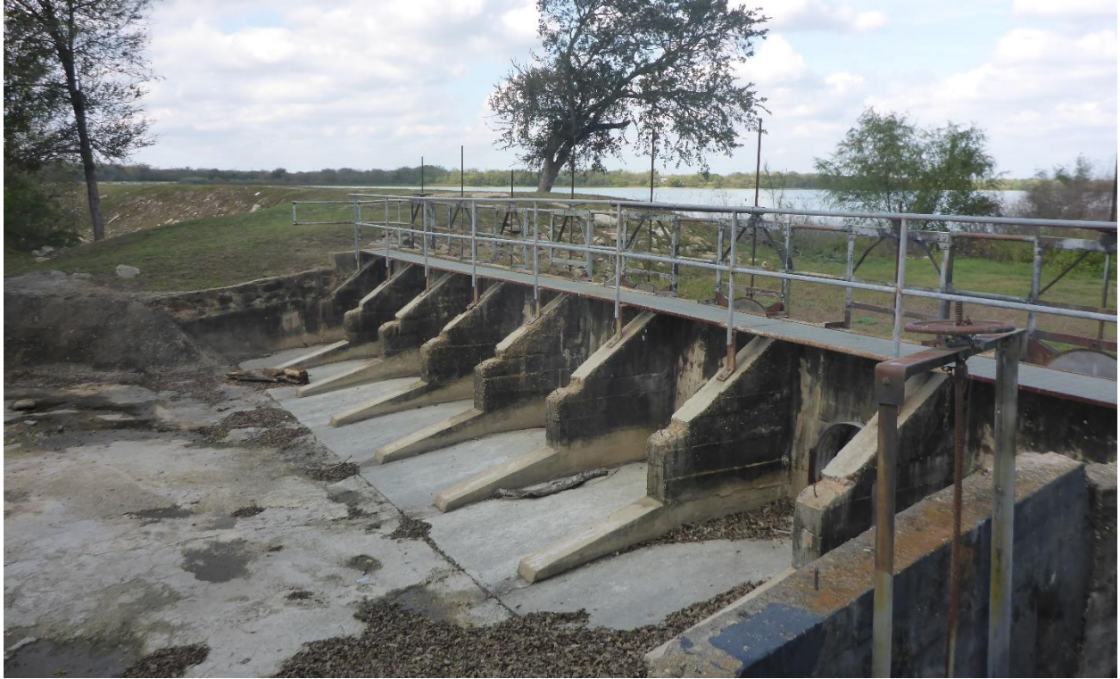
Photo 11: Spillway Downstream Face and Channel (Looking right)
