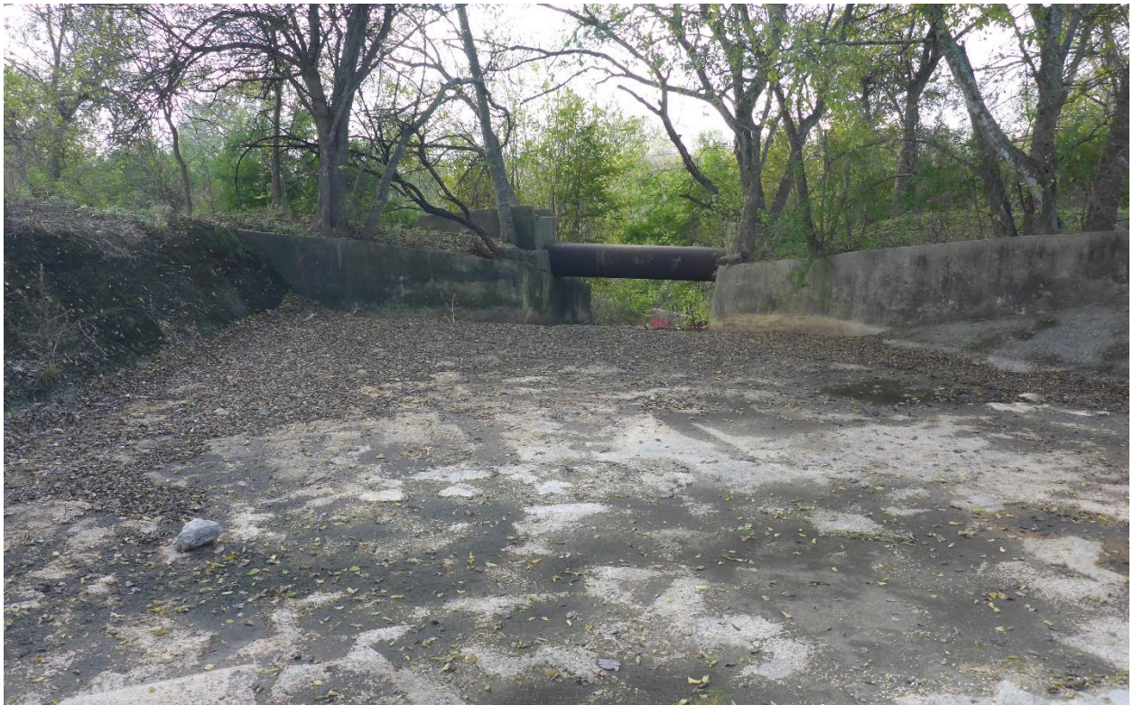
Photo 14: Spillway Channel Looking Downstream
