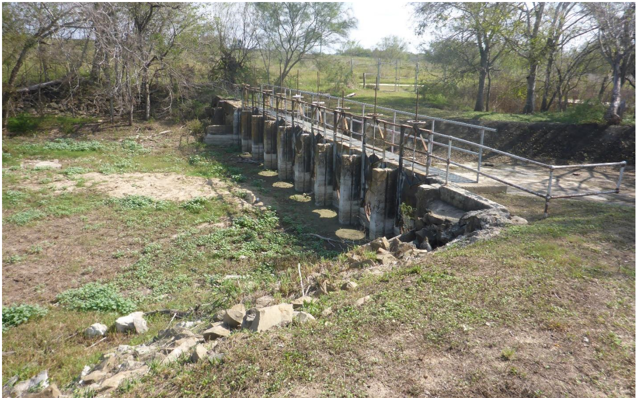
Photo 8: Spillway (Looking left from upstream)
