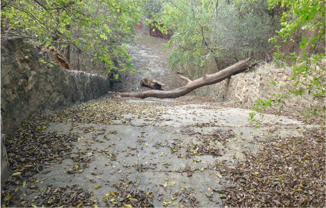
Photo 15: Spillway Channel Looking Downstream
