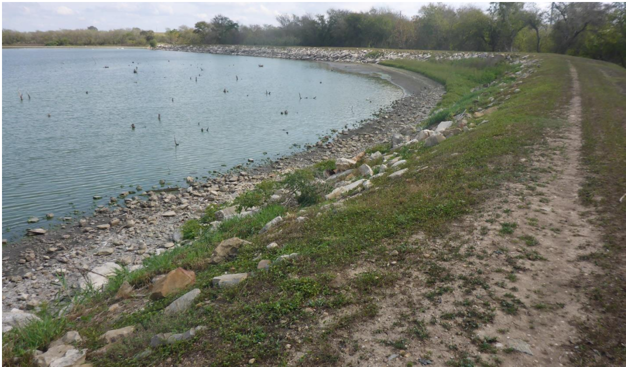
Photo 4: Upstream Embankment Slope
