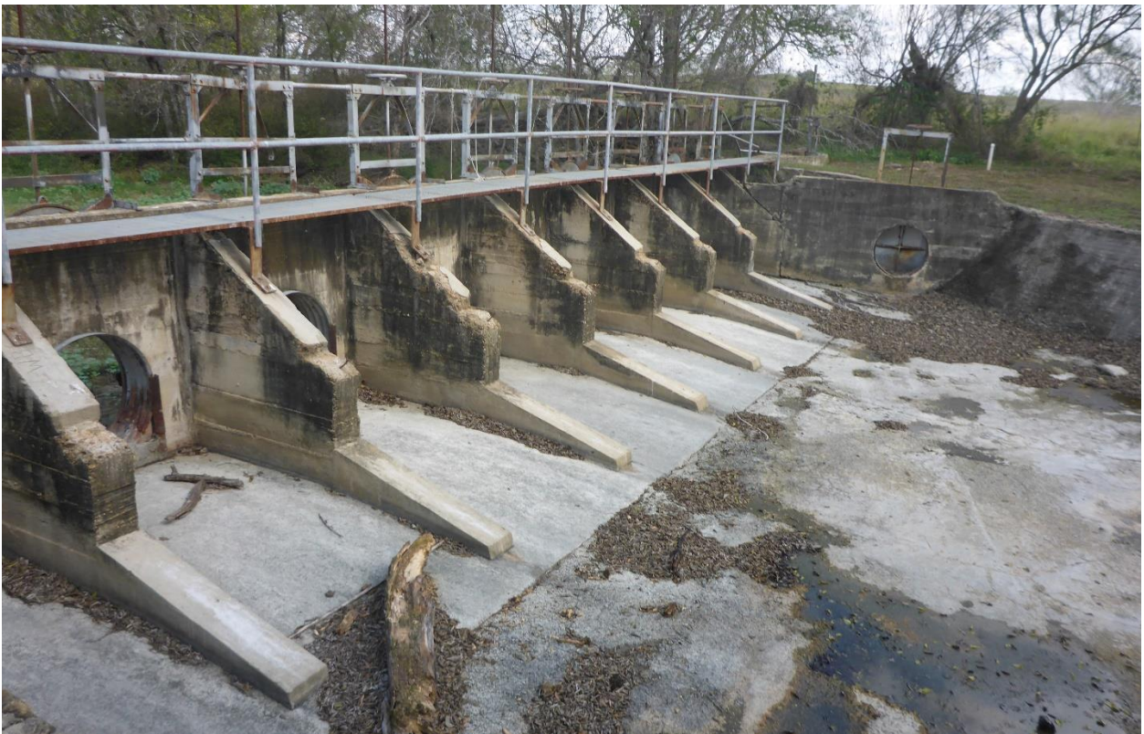
Photo 10: Spillway Downstream Face and Channel (Looking left)
