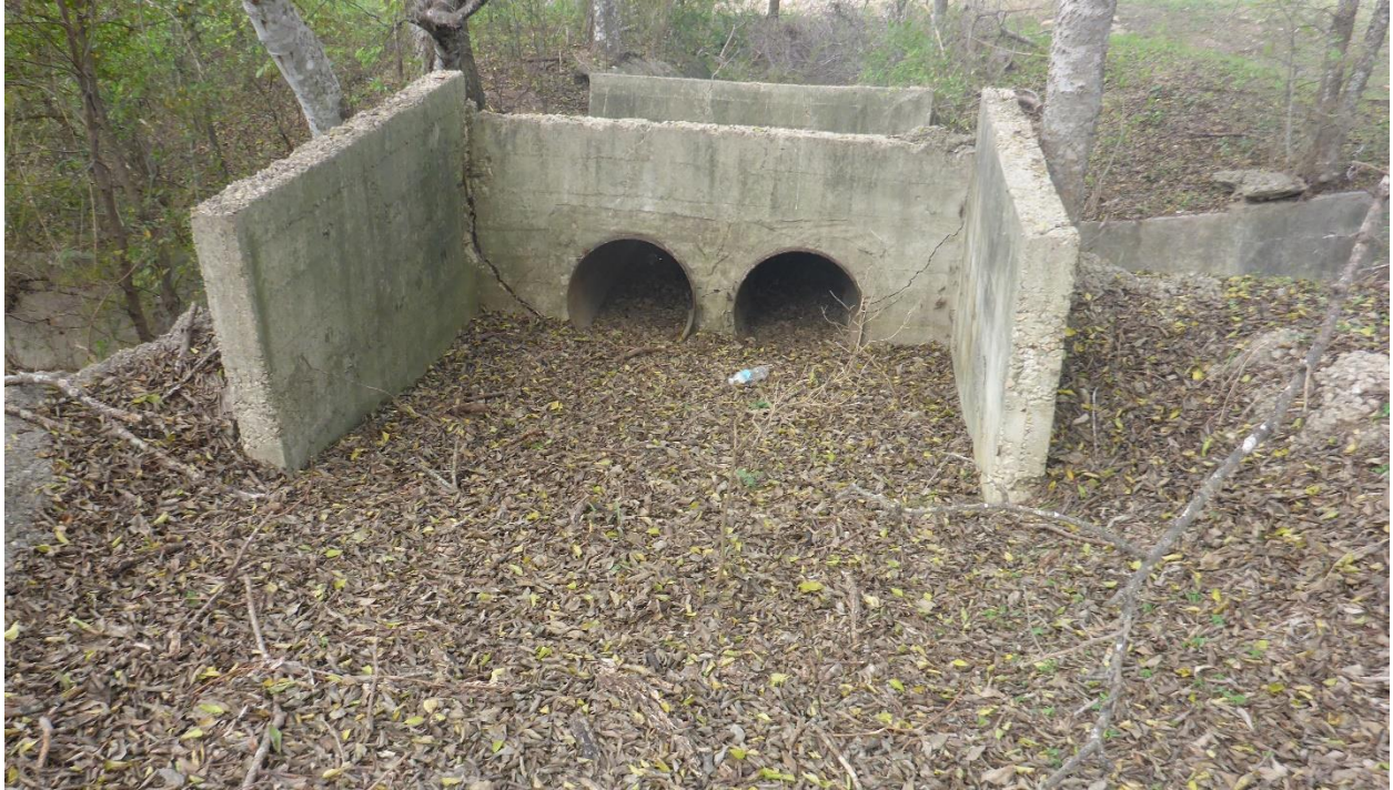
Photo 13: Irrigation Culvert Crossing over Spillway Channel
